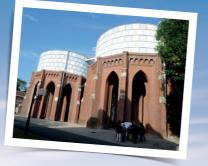
textile mills for water, both towns had those tanks built. The engineer Varennes was asked to design them and had the first tanks of water for industrial purposes in the Lille metropole area erected in 1863. Both brick constructions are topped by an open tank made of riveted cast iron. The water was drawn from the river Lys. This project was one of the first jointly initiated by Tourcoing and Roubaix. The tanks were restored by the Water Company of Northern France in 1989 and 1990.
